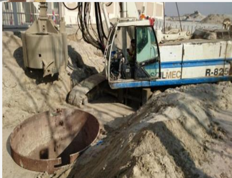
SOILMEC R825 WITH DOUBLE ROTARY
